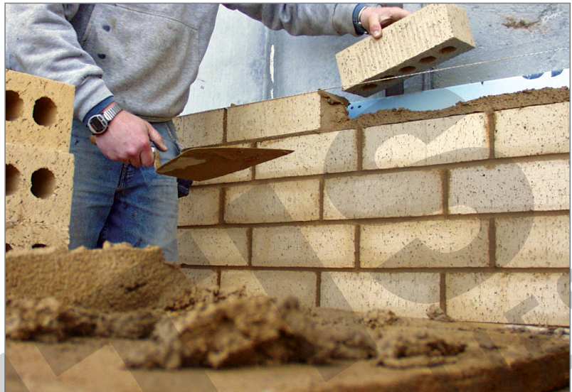
Consistent custom colored mortar, every time
