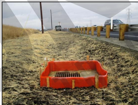
Road Construction – Roadside Ditch
