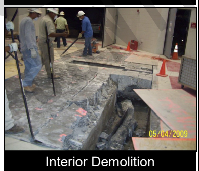
Concrete Demolition
