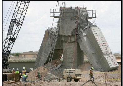
Demolition of Highway Bridge
