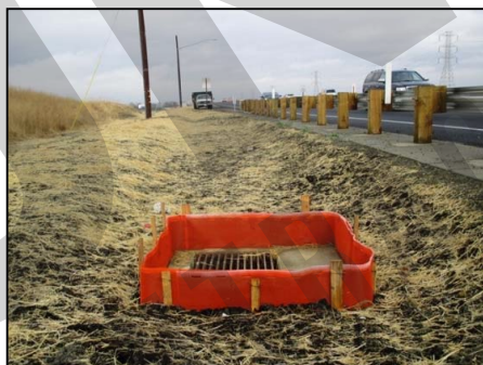
Road Construction – Roadside Ditch
